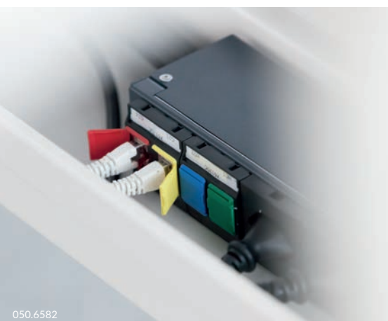
Custom-made by R&M for Swiss Re Next: compact DDS outlets in the desks.
