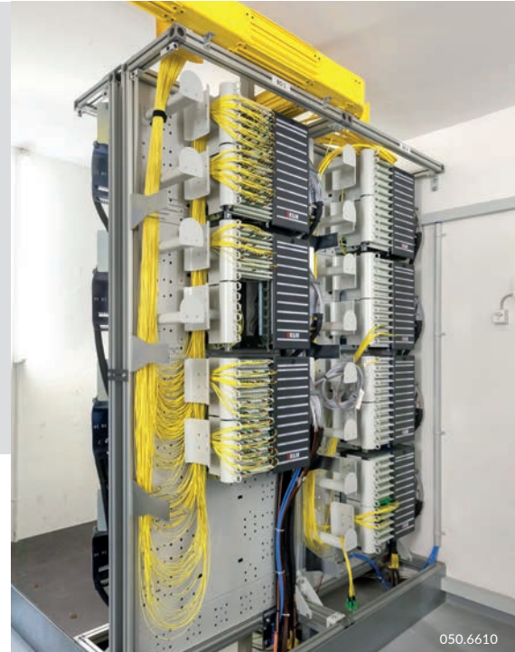
Distribution center with the R&Mfoxs system: Among other things, 311.5 km of micro cable with 12-72 fibers as well as 35.5 km of feeder cable with 288-576 fibers were used
