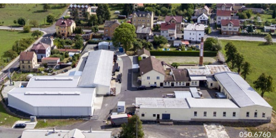
The R&M cable plant in Děčín, in the north of the Czech Republic
