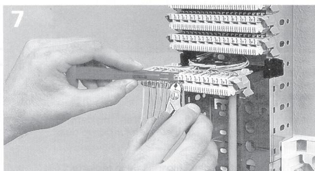
■ If wiring with a Tooly, the wires have to be cut with a diagonal cutter after insertion into the wire baffles, and then wired.
