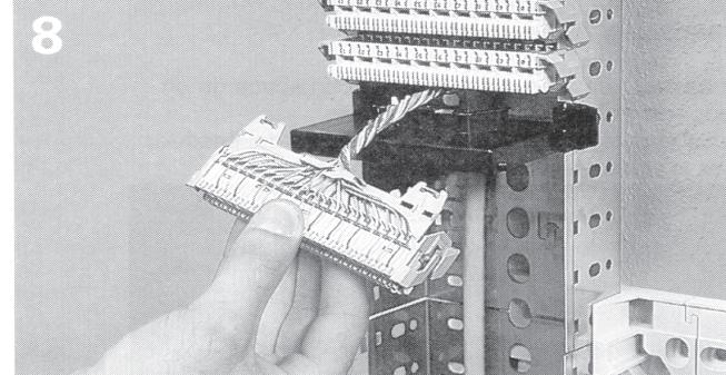
■ Remove the module from the wiring base and loosen the cable reserve.
