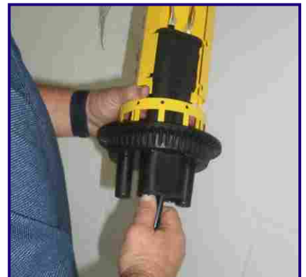
42 Enter the cablegrip into port.
