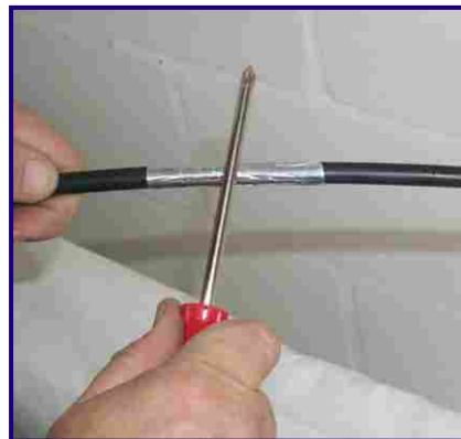
14 Smooth out aluminium tape with a suitable tool. (Not required when using a rubber cablegrip)
