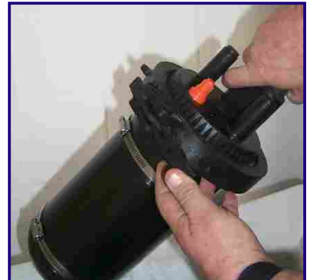
33 Tighten the clamp to seal (To re-enter, loosen clamp and remove cover).
