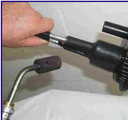
31 Shrink heatshrinkable sleeve down onto cable. Allow to cool. (Not required when using a rubber cablegrip)
