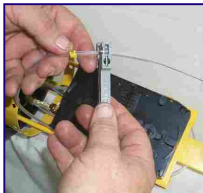
26 Cut the tube carefully with a suitable tool as not to damage the bare fibres.
