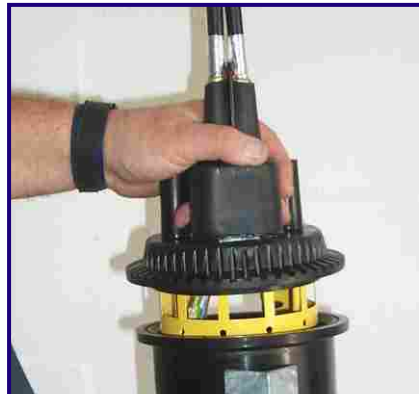
32 Check that the 'O' Ring is not damaged, free from any dirt and seated properly. Fit cover onto the closure
