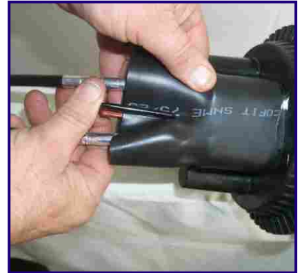
30 When using oval port, separate cable and insert branch clip. (Not required when using a rubber cablegrip)
