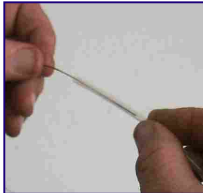
23 Feed transportation tube over bare fibres up to cable sheath opening “B”. Not applicable if fibre tube is not cut.
