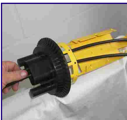
34 The following steps are to be followed when using the cablegrip: Pass cables through the selected port leaving sufficient cable for splicing. Prepare cables in accordance with standard jointing practice.
