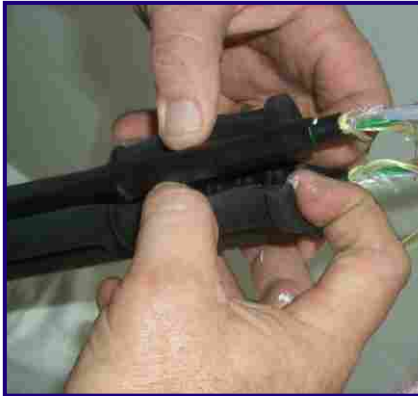
37 Fit cables into split cablegrip.
