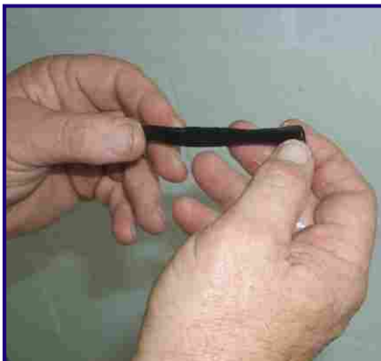
40 Cut a strip of mastic tape 5mm x 100mm.
