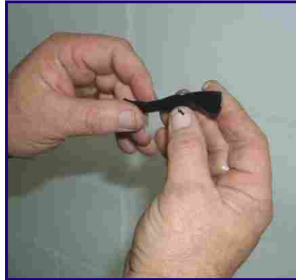
38 Cut mastic tape 10mm x 70mm and fold over double.
