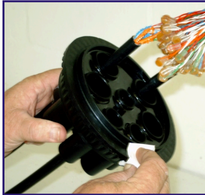
20 Clean and inspect the seating surfaces of the base and the cover for any damage.
