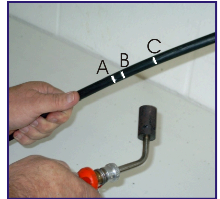
12 Flame brush the cable sheath between B and C.
