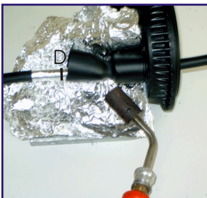
16 Position the cable with the aluminium tape \pm 20 mm (B to D) inside the heatshrinkable sleeve and shrink down onto cable. Allow to cool down completely.
