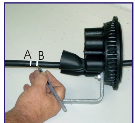
9 Mark the cable B \pm 20 mm from A towards the heatshrink.
