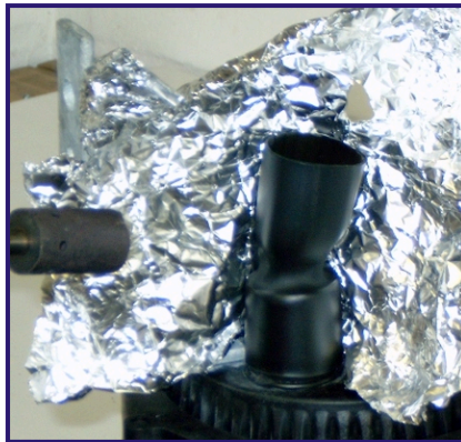
5 Place the heatshrinkable sleeve over the open port and shrink down onto port, leaving \pm 10 mm unrecovered at the end of the port.
