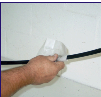
7 Clean the cable sheath to length required. Prepare cable for jointing in accordance to standard jointing practice. Pass the prepared cable through the open port, leaving sufficient cable for jointing.
