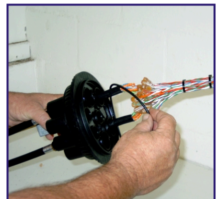
18 On completion of jointing remove "O" ring from the closure base.
