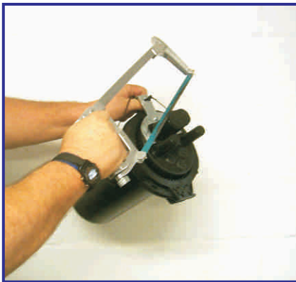
1 Remove closure from packaging, select required cable entry port and open with a suitable tool.
