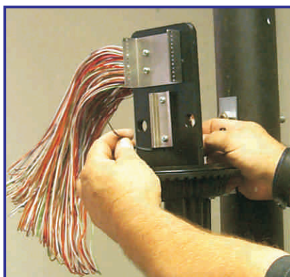
17 Secure the cables to the support frame with the cable ties. Position the closure and secure mounting bracket.
