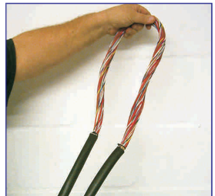
6 Remove cable sheath and prepare the cable according to standard jointing practise.
