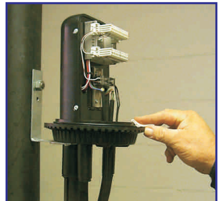
33 Closing: Make sure all sealing surfaces and O ring are clean and undamaged.
