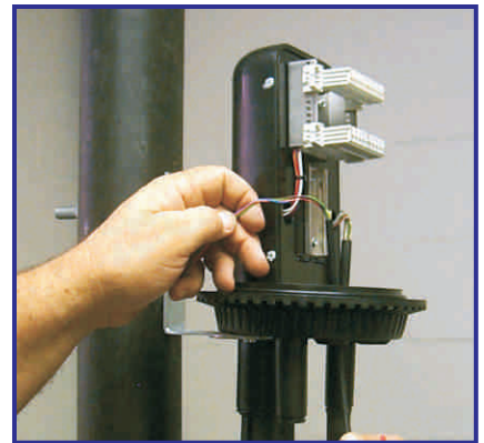
30 Pass the Dropwire through the pierced hole leaving sufficient cable for terminating. Prepare the cable according to standard jointing practise and terminate, fit IDC connect module if required.
