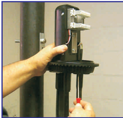
29 Entry for Dropwire (2 pair): Pierce a hole through a selected 4 x 5mm rubber grommet with a suitable tool.
