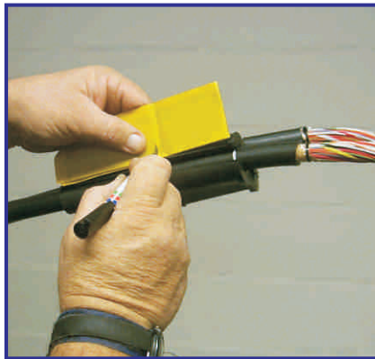
11 Measure, mark and cut the mastic tape, 4 pieces of \pm 18\text{mm} \times 75\text{mm} .
