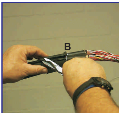
14 Trim off the excess mastic tape. Repeat steps 11 to 14 for the second cable.
