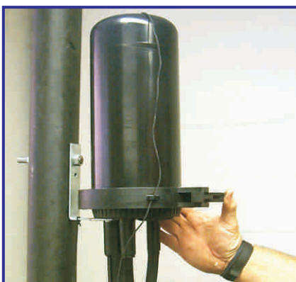
34 Replace closure body, fit and secure swing clamp. (The closure body and the swing clamp are secured to the Closure Mounting Bracket by a UV stabilised nylon cord).
